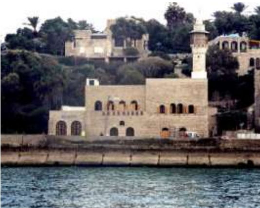
Image 15 Mina Mosque renovated
