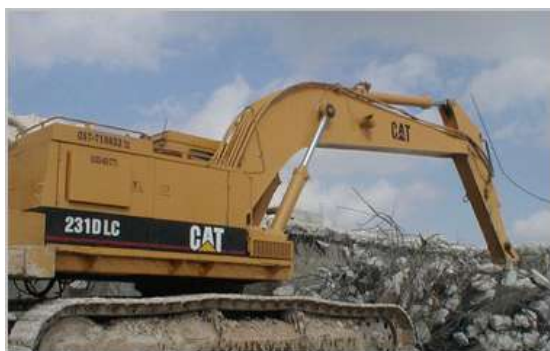
Image 20 Bulldozing a house
